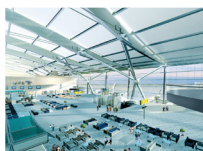
Terminal 5 Heathrow airport (T5) – London (Express group & Laing O'Rourke JV)
