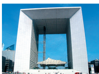
Arche de la Défense Paris (Cutting and bending: Breteuil armature in France, Fixing : SPATP/SPATB)
